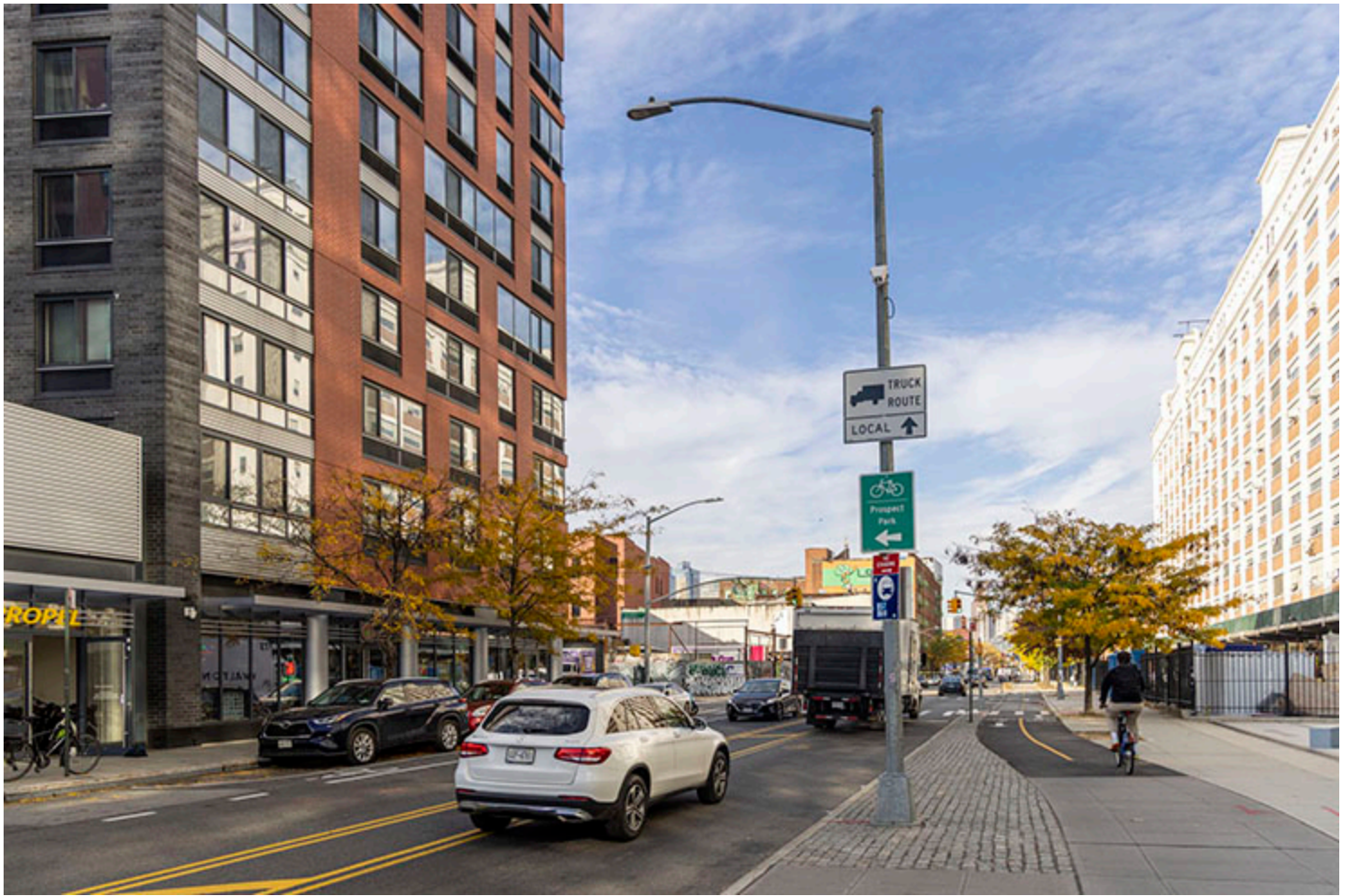
A street activity sensor mounted on a streetlight along Flushing Avenue in Brooklyn.
