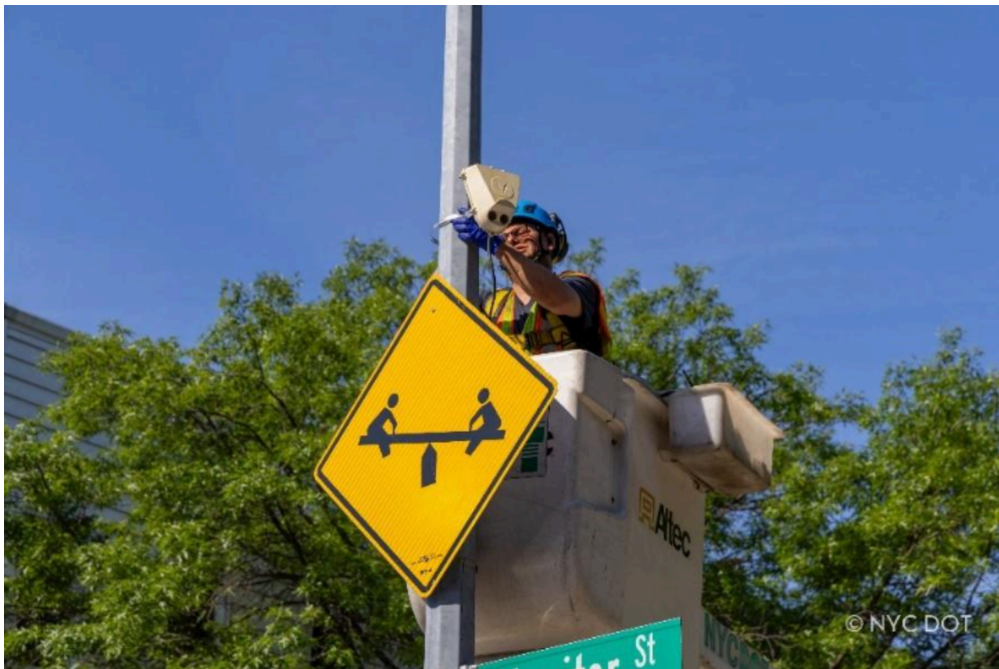
NYC DOT Traffic Operations worker installing a new activity sensor in Greenpoint, Brooklyn.
